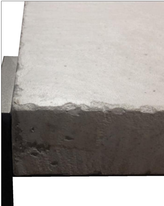
Béton 350 / Concrete 350 / Cemento 350
